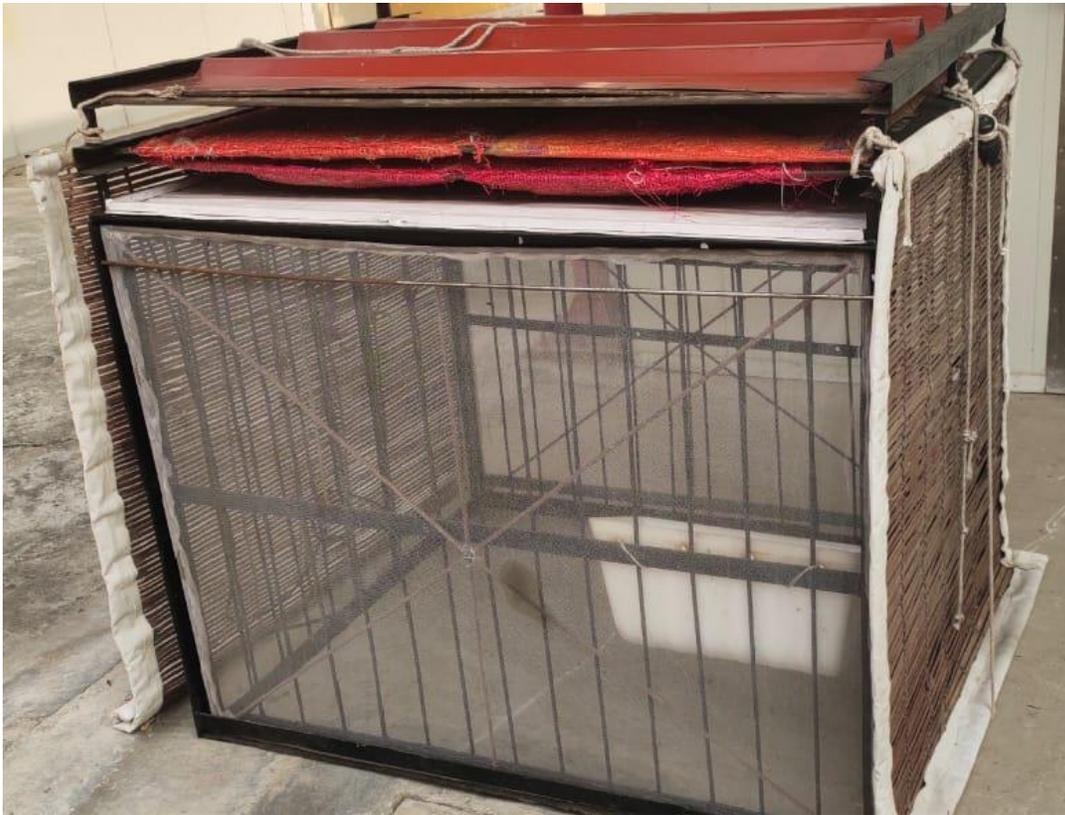
**Figure 2.** Livestock housing module fixed with flies proof nylon mesh for hot humid season
